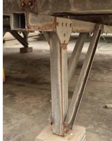
The real case in Changbin Industrial area in Taiwan. The mounting serious corrosion just after four years.
